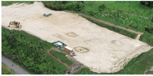
Fig.2 Bird's-eye view of the environmental site in Kyushu University.
