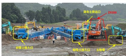
Fig. 9 Overview of the First On-Site Application Experiment
