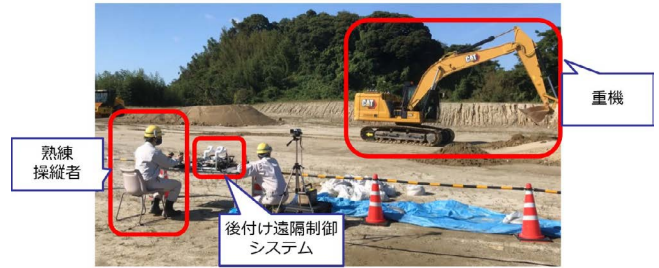
Fig.9 The experiments using the backhoe operated by the proposed system.
